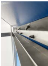
Carpentry made of AISI 034 stainless steel
