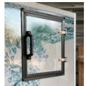
Inspection hatch for ice area
